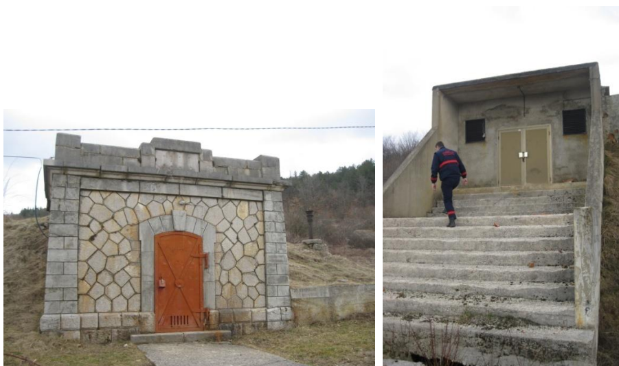
Figure 4 and Figure 5: Reservoirs „Novakovići“ ( V=200 \text{ m}^3 ) and „Bursaći“ ( V=2000 \text{ m}^3 )
